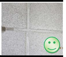
Discuss the masonry joints...They need to be full, properly tooled (<u>compressed</u> in the joint, either flush or concave)...We do not want the joints to have voids or mortar sticking out of the joint, creating ledges and improper membrane thicknesses at these irregular shapes, potentially creating failure in the AVB system.
