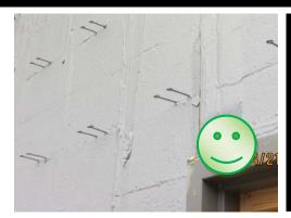
Talk about the wall ties and the need to have them straight and level...if the wall ties are bent, during the unbending, the AVB membrane will tear and will create a breach in the membrane system, potentially creating failure in the AVB system.
